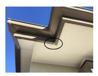
Fascias Replace fascia joiner to match correct Minor Defect Type: F colour
