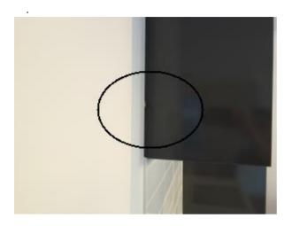
Cupboards Adjustment of all cupboard doors and Minor Defect Type: F drawers required
