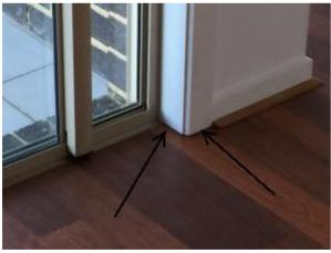
Built in robe Incomplete installation Minor Defect Type: F
