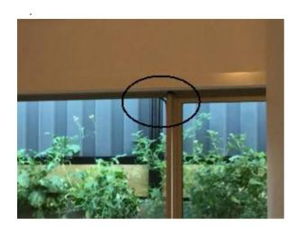
Doors and frames Sand back and repaint damage Minor Defect Type: A section of bedroom three door
