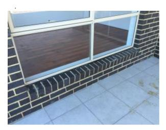
Sills Removal of excess mortar under brick Minor Defect Type: F sill is required
