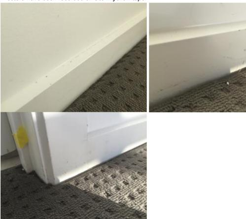
Walls Excessive gaps to underside of door Minor Defect Type: F jambs/architraves
