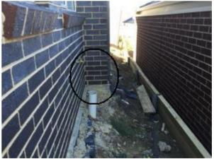
Slab and wall location Slab or wall installed to incorrect Further Investigation Type: F location
