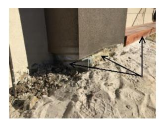
Walling Staining to rendered wall – re-painting Minor Defect Type: F required
