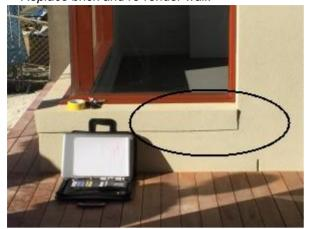
Doors Timber in contact with the ground Minor Defect Type: F susceptible to decay
