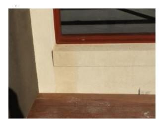
Walling Sub-standard render application Minor Defect Type: F
