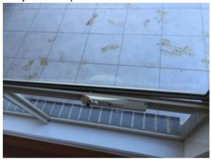
Windows Damaged window frame Minor Defect Type: A
