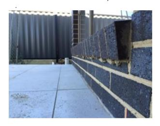
Doors Bowed door sill to replaced Minor Defect Type: A, B Replace brick sill to enable timber sill tobe placed level across the brick sill.
