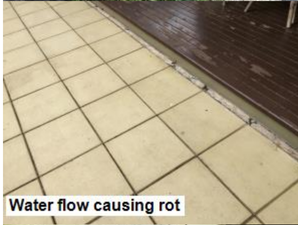
evidence of water flow under the home view from the south elevation
