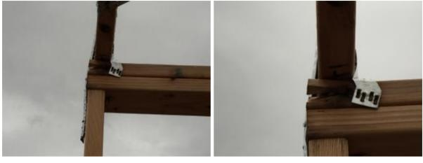
WindowsHorizontal bow to windowMinor DefectType: FInadequate gauge in material over that particular span.Replacement recommended.
