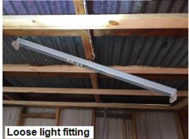
Unsafe electrical installations
