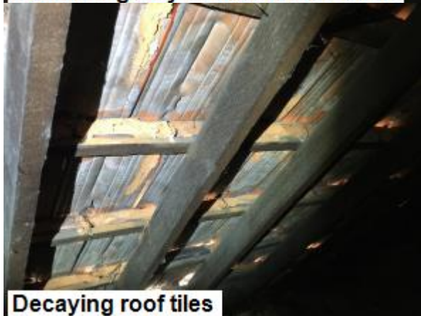
Powdering clay roof over insulation
