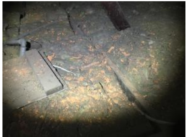
Powdering clay roof over insulation
